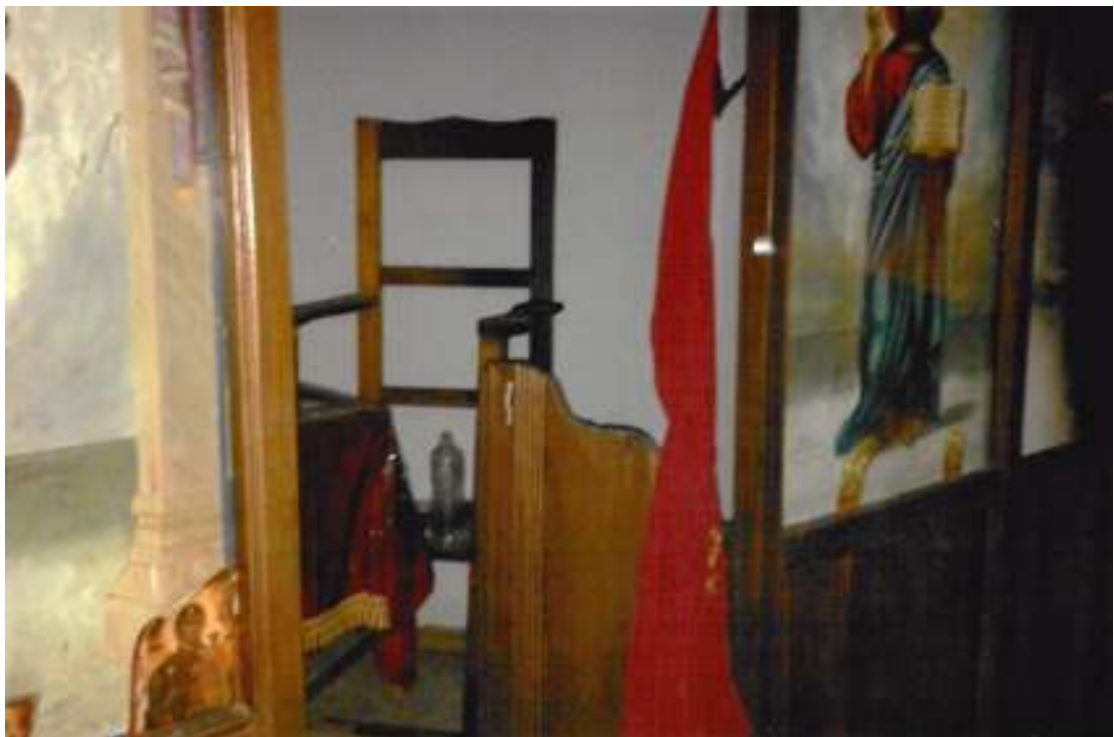
Damage caused by the fire
